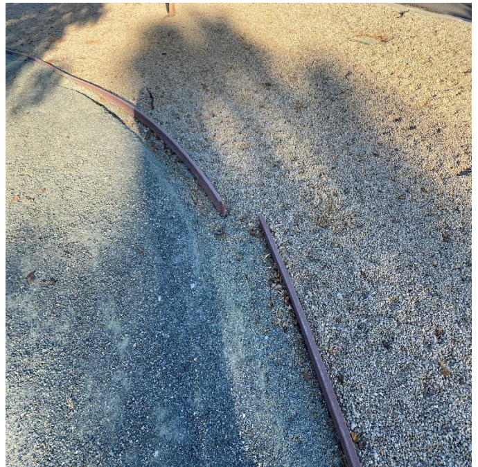
Edging is warping and bending due to sun/heat and needs re- staking
