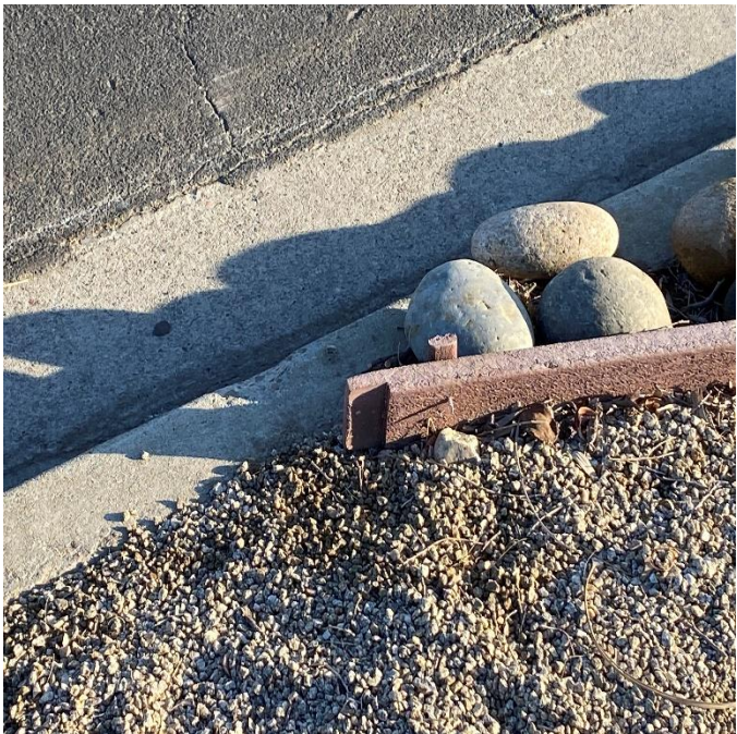
Edging is warping and bending due to sun/heat and needs re- staking
