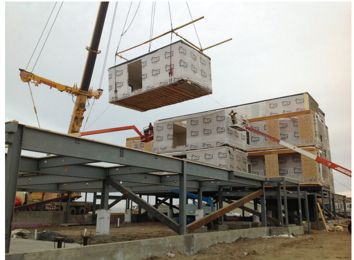
Full Height Support Structure using a steel foundation on concrete piers.
