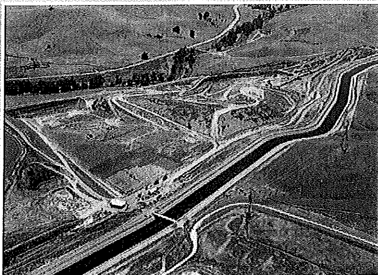
An active landfill situated adjacent to a canal in Clovis. The section on the left has been lined while the waste on the far right is being mined to rebuild the disposal unit with a liner.
