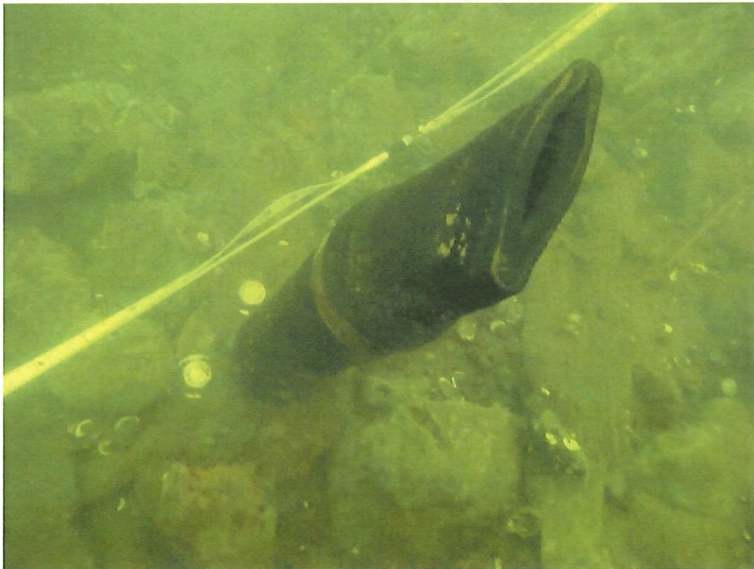
Photo 12 – Diffuser #28, Post-Cleaning
