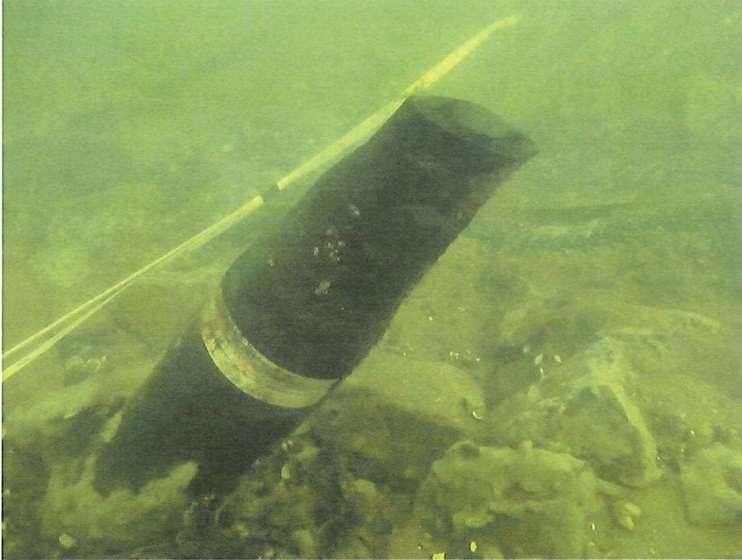
Photo 13 – Diffuser #31, Post-Cleaning
