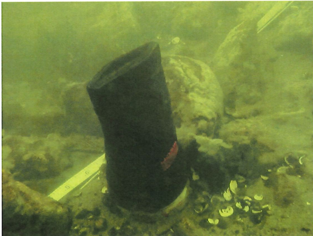
Photo 2 – Diffuser #1, Post-Cleaning
