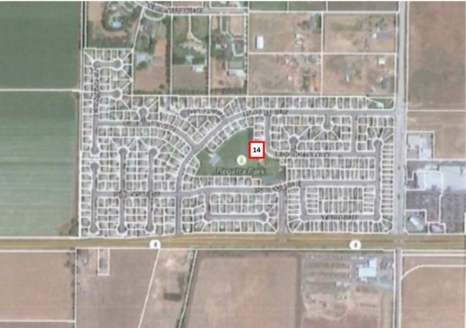
14 Lift Station "S" (North edge of Regatta Park-Foghorn Way)
