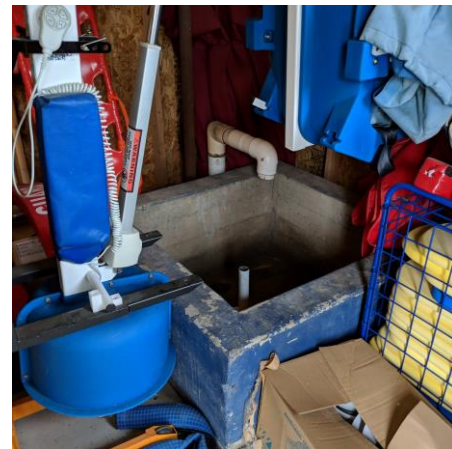
Photo #4 View of the backwash pit and stored ADA lift
