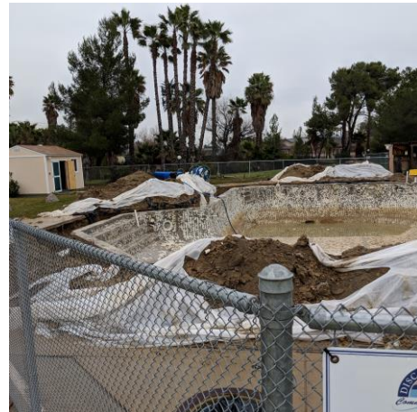
Photo #2 View of the shallow end of the pool
