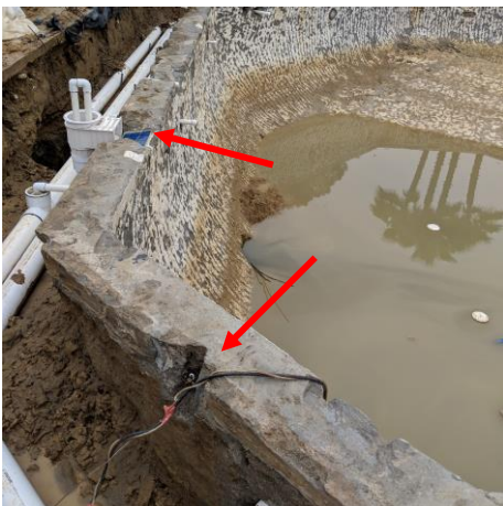
Photo #5 View typical new piping, skimmers, and bonding
