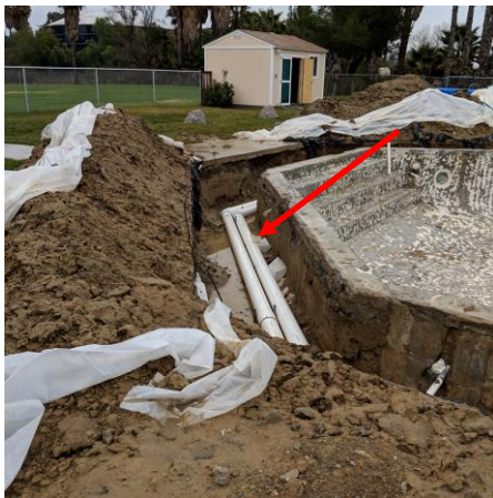
Photo #3 View of trench drains around the stairs
