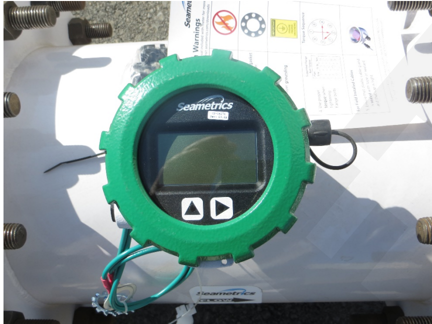
Figure 3 - Magnetic Flow Meter
