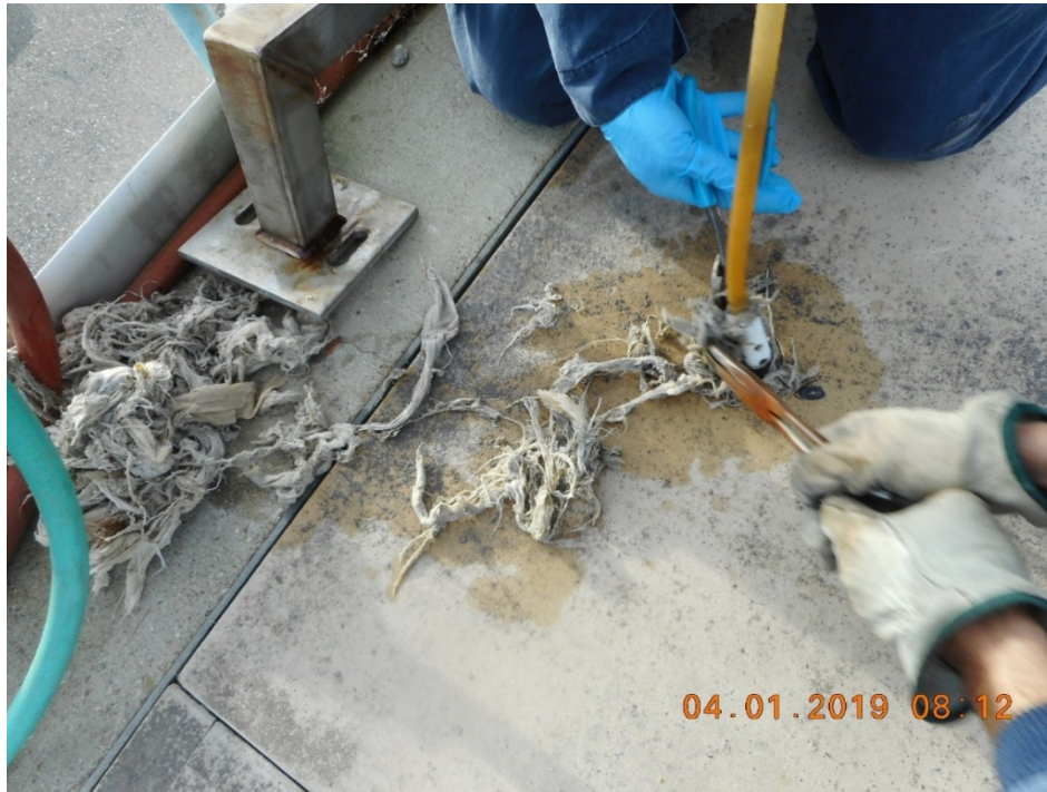
Figure 5-12 Rags Being Removed from Portable Sampler Intake Strainer on 4-1-2019
