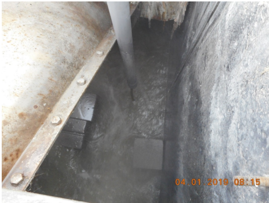
Figure 5-13 Initial Configuration of Concrete Blocks and Sampler Intake Tube in Screen Channel on 4-1-2019
