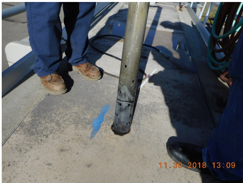
Figure 5-9 Perforated Pipe Surrounding Sampler Intake Strainer
