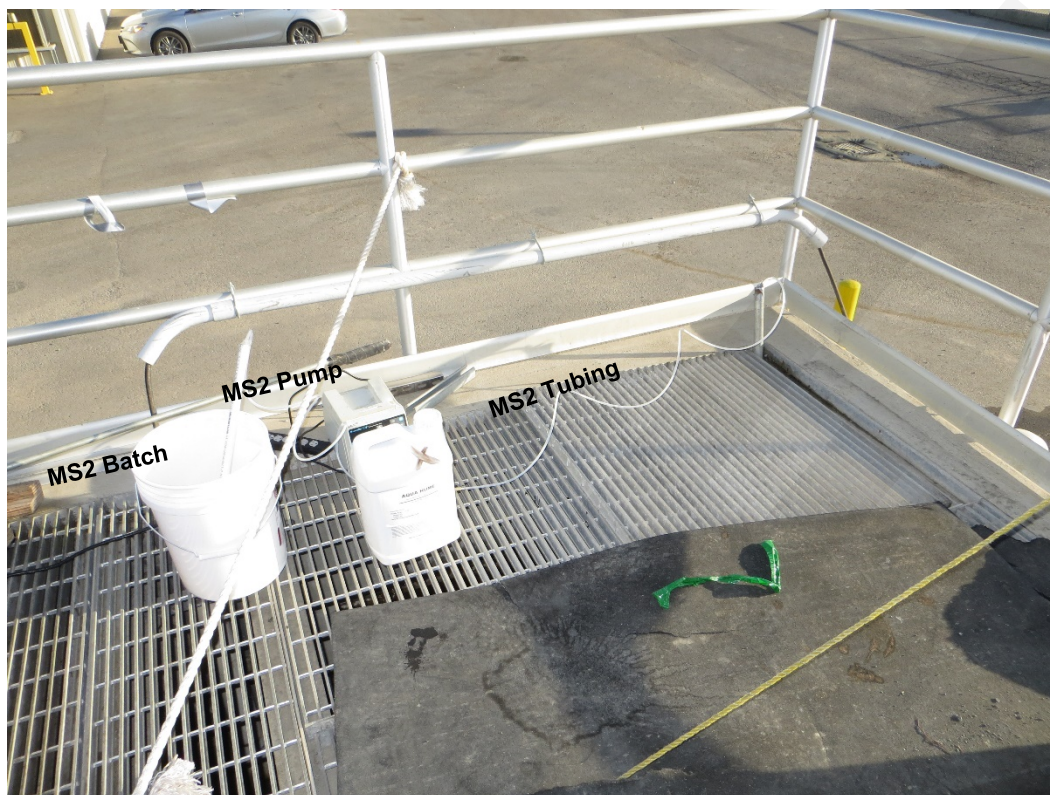
Figure 2 - MS2 Injection Point (Recirculation Suction Piping Below)
