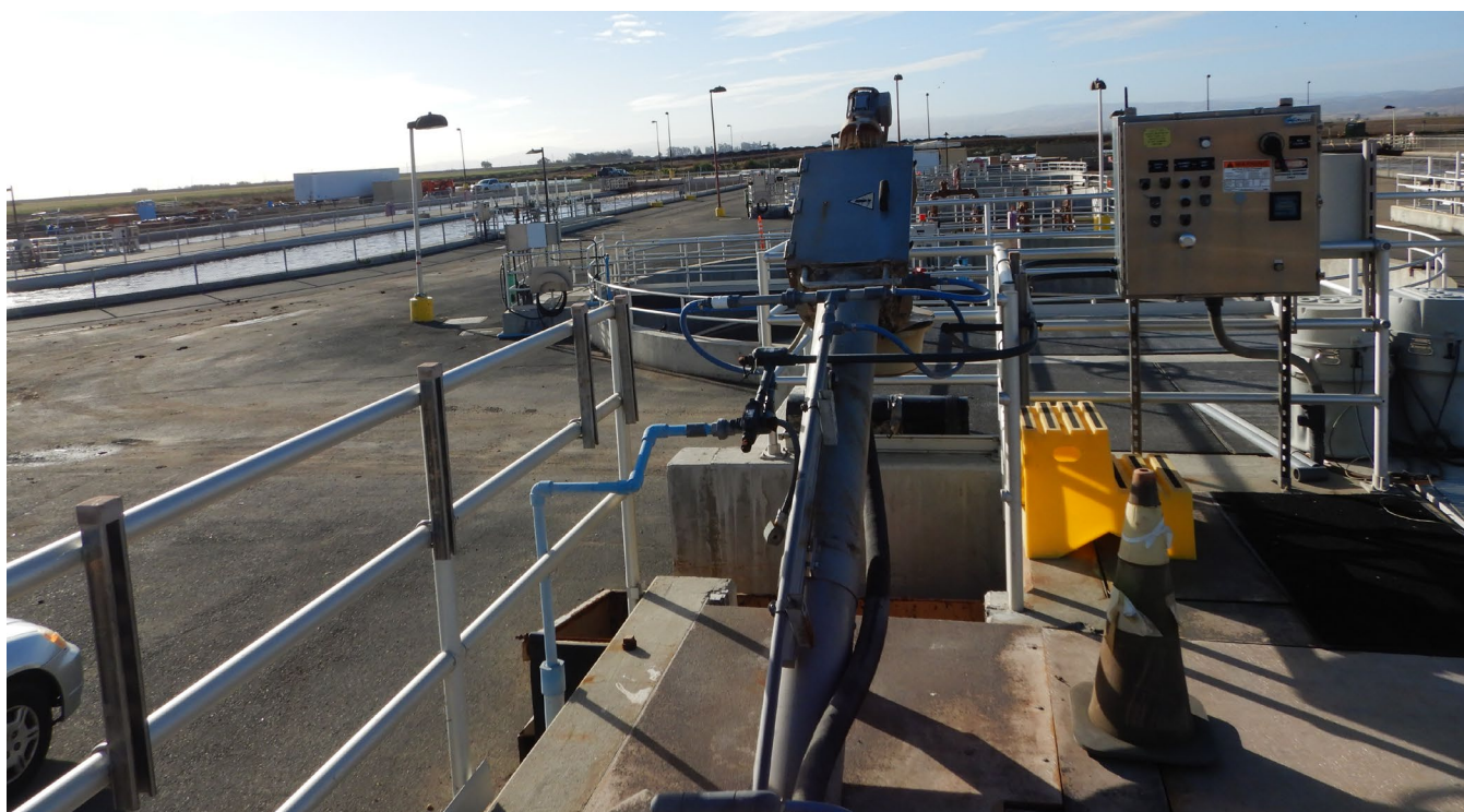
Figure 1: All influent flow is sent to Plant 2. Plant 1 is currently not in operation. The Magnetic influent flow meter measures flow coming from Plant 1. The flow meter is used for internal process control and as a backup in case the Parshall Flume goes off-line.
