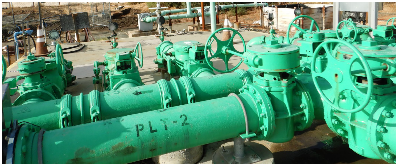
Figure 1: All influent flow is sent to Plant 2. Plant 1 is currently not in operation. The Magnetic influent flow meter measures flow coming from Plant 1. The flow meter is used for internal process control and as a backup in case the Parshall Flume goes off-line.
