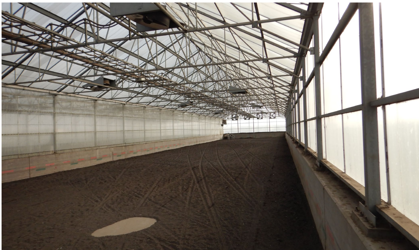
Figure 8: One of the four active solar dryers.
