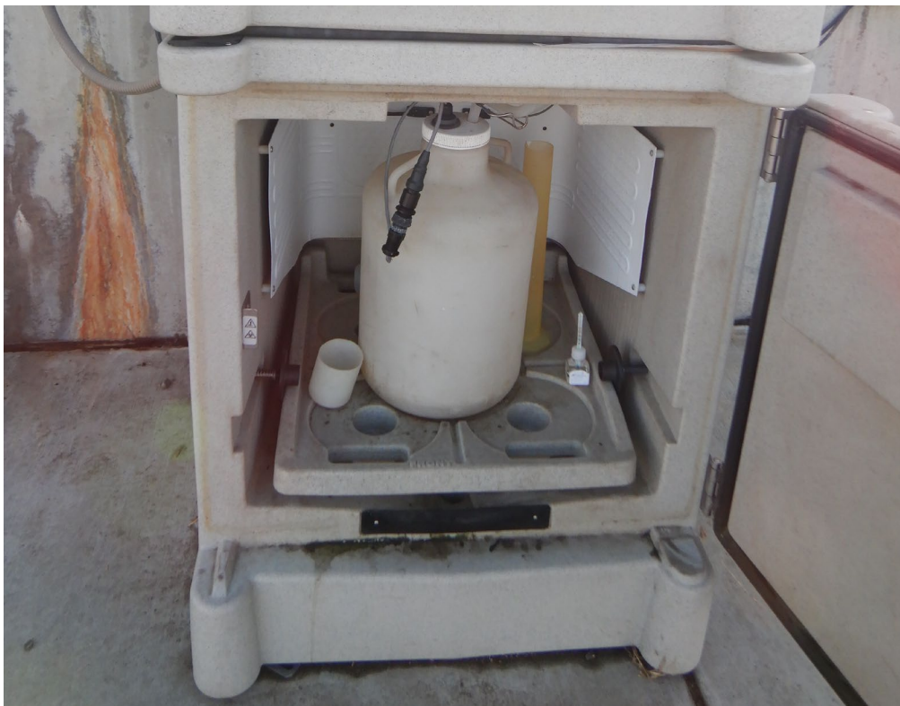
Figure 10: The influent composite sampler had an internal temperature of 3.0°C.
