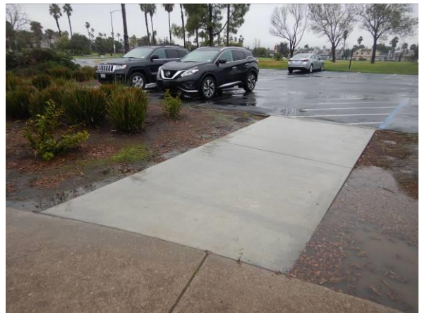
Photo #6 Typical concrete pavements.
