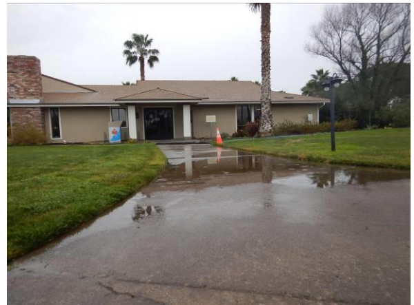
Photo #22 Overview of approach to building. Notwithstanding water in localized areas.
