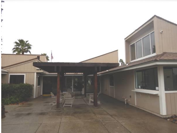
Photo #33 Partial east building elevation.
