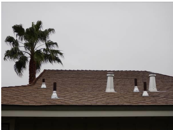
Photo #47 The roof consists of asphaltic composition shingles and skylights.
