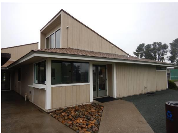
Photo #35 Overview of ADA accessible entrance provided at the north building elevation.
