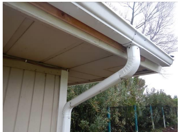
Photo #48 Typical gutter and metal downspout.
