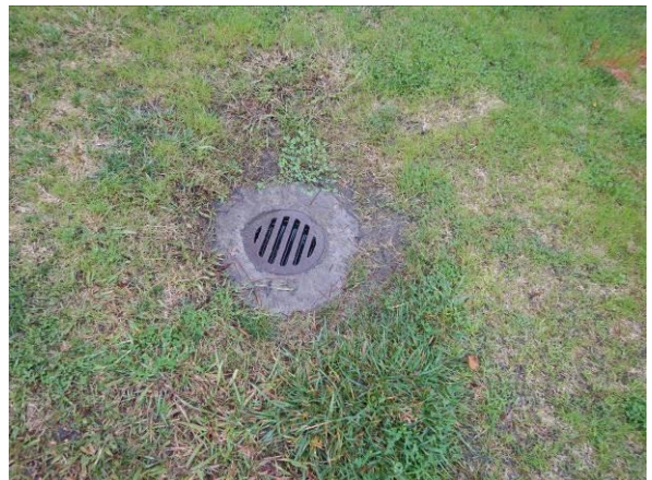
Photo #28 Typical area drain in landscaped area.
