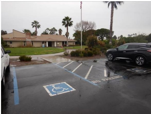
Photo #81 Accessible parking stall. Note missing vertical signage.
