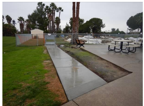
Photo #18 Chain-link fencing temporarily encloses the pool area currently under construction.
