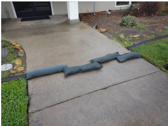
Photo #23 Property management placed sandbags in front of the main building entrance in an attempt to mitigate water intrusion into the building.
