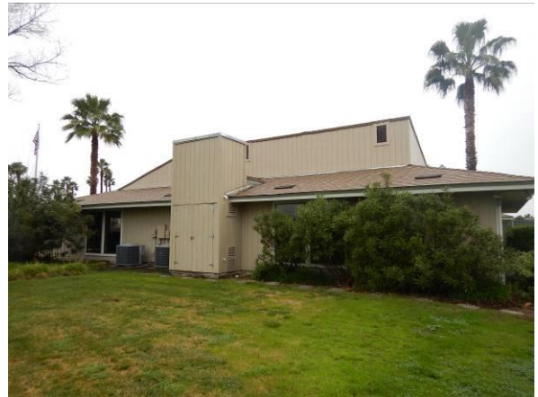
Photo #32 Overview of south building elevation.
