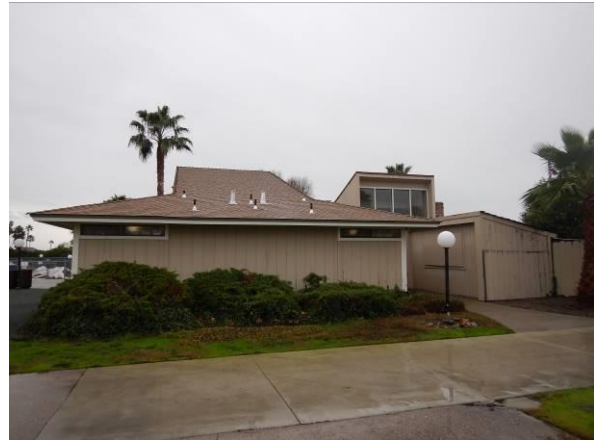
Photo #34 Partial north building elevation.
