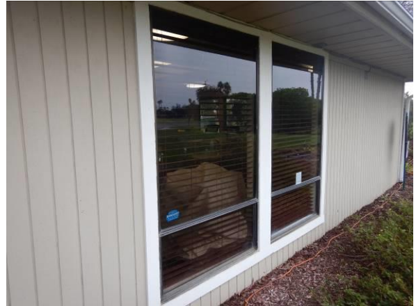
Photo #38 Typical window unit.
