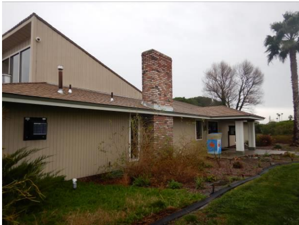
Photo #31 Overview of west building elevation.
