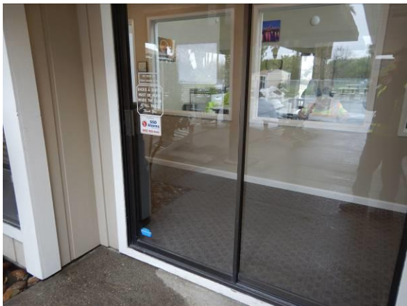
Photo #41 Sliding glass door at the east building entrance.
