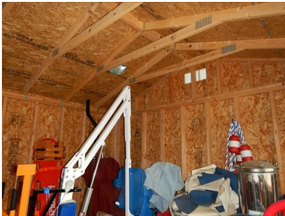
Photo #21 Storage shed interior.
