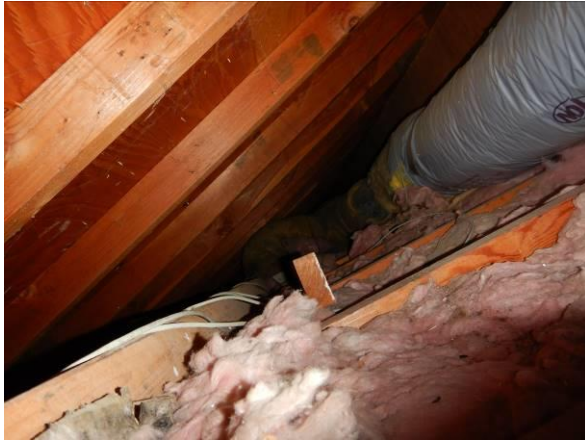
Photo #37 Overview of typical wood-frame building construction, as observed from attic
