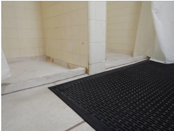
Photo #61 Close-up view of shower entrance threshold. Women's is similar.
