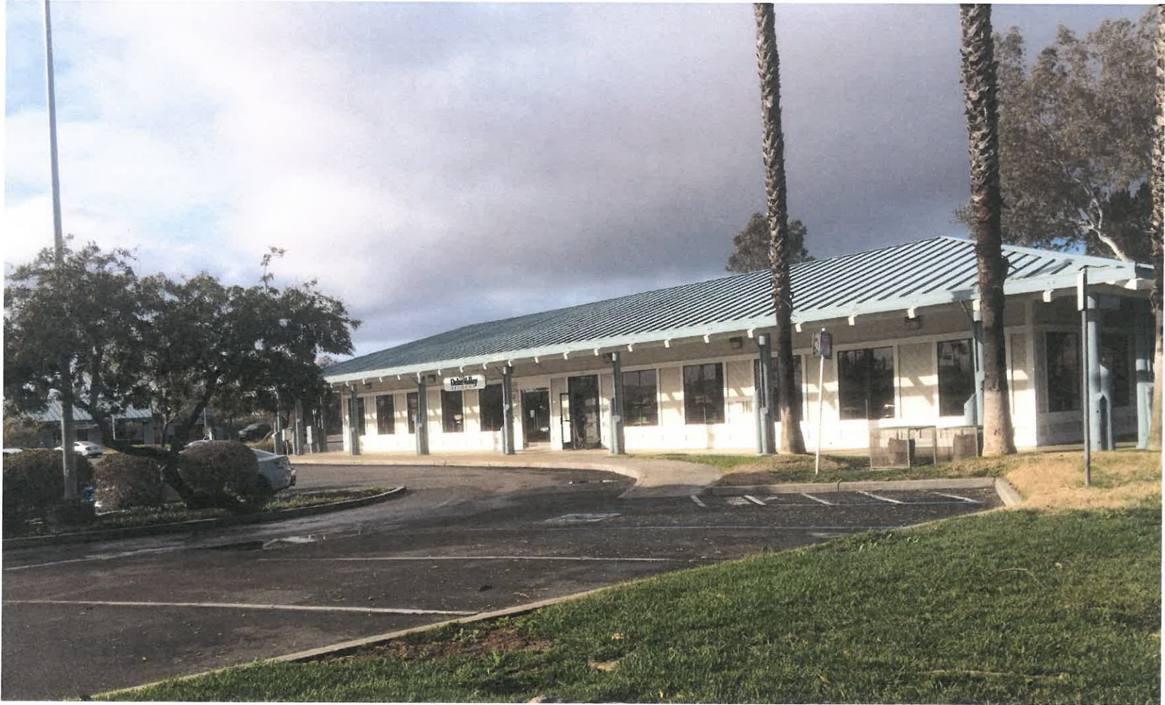
View from Discovery Bay Blvd of building at 1520 Discovery Bay Blvd January 26, 2016
