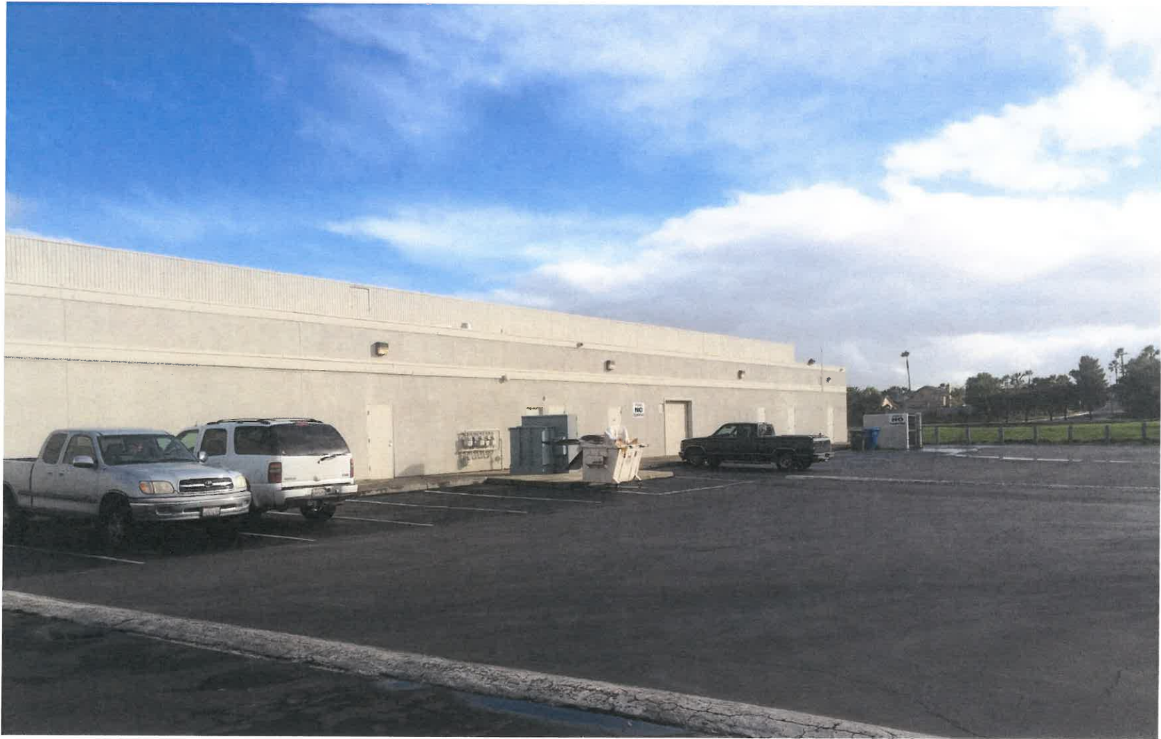
View of parking behind building at 1540 Riverlake Rd January 26, 2016
