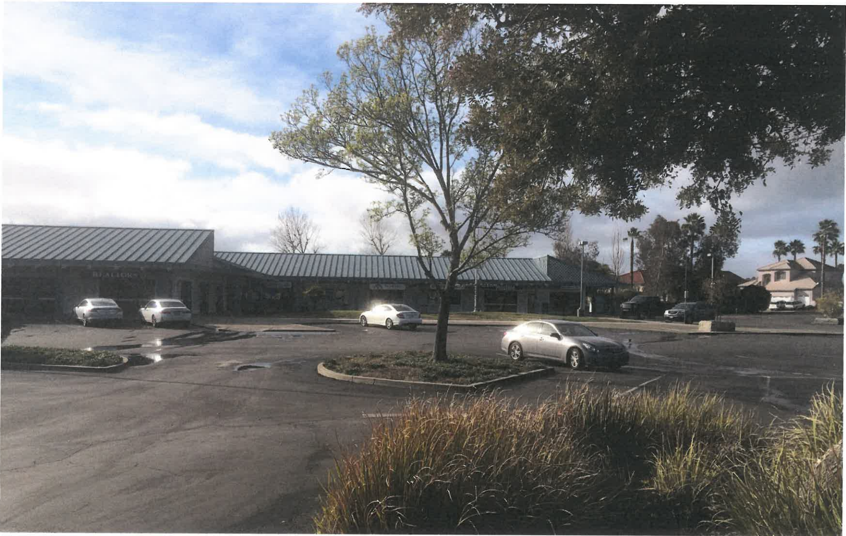
View from building at 1520 Discovery Bay Blvd toward building at 1555 Riverlake Rd January 26, 2016
