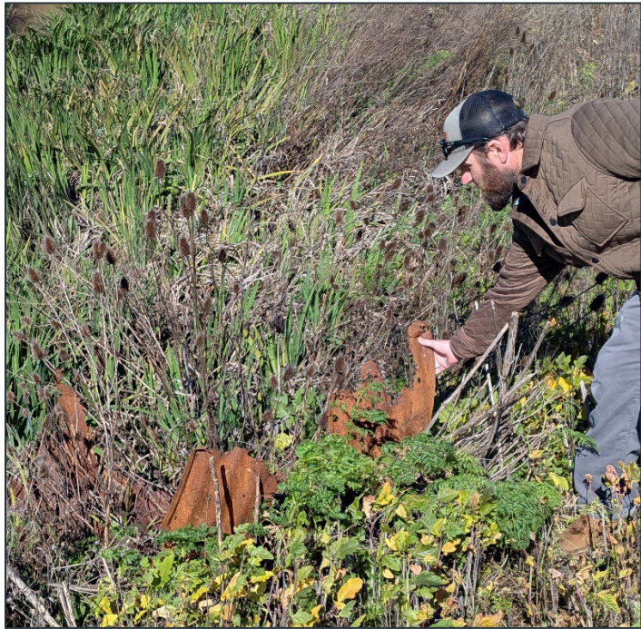
Figure 4: CMP Culvert Pieces
