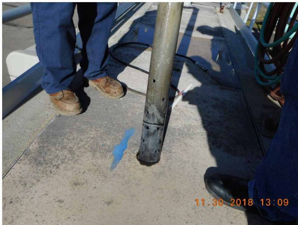
Figure 5-9 Perforated Pipe Surrounding Sampler Intake Strainer
