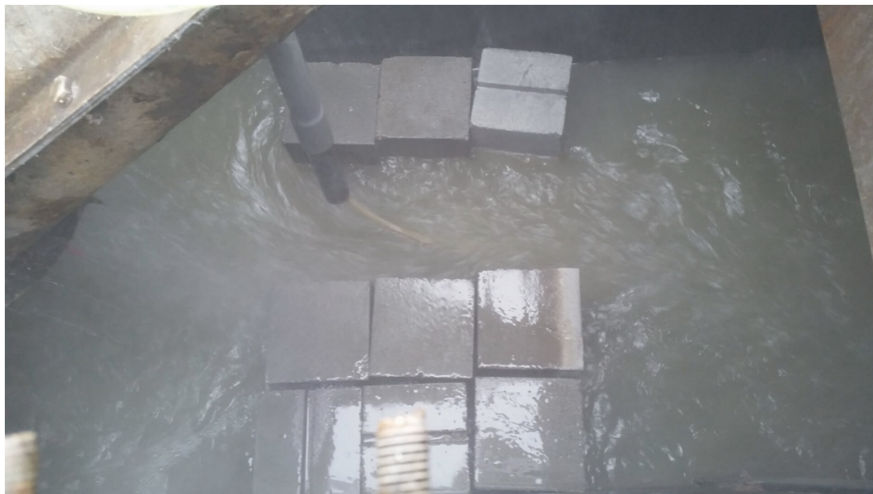
Figure 5-14 Final Configuration of Concrete Blocks and Sampler Intake Tube in Screen Channel on 4-4-2019.
